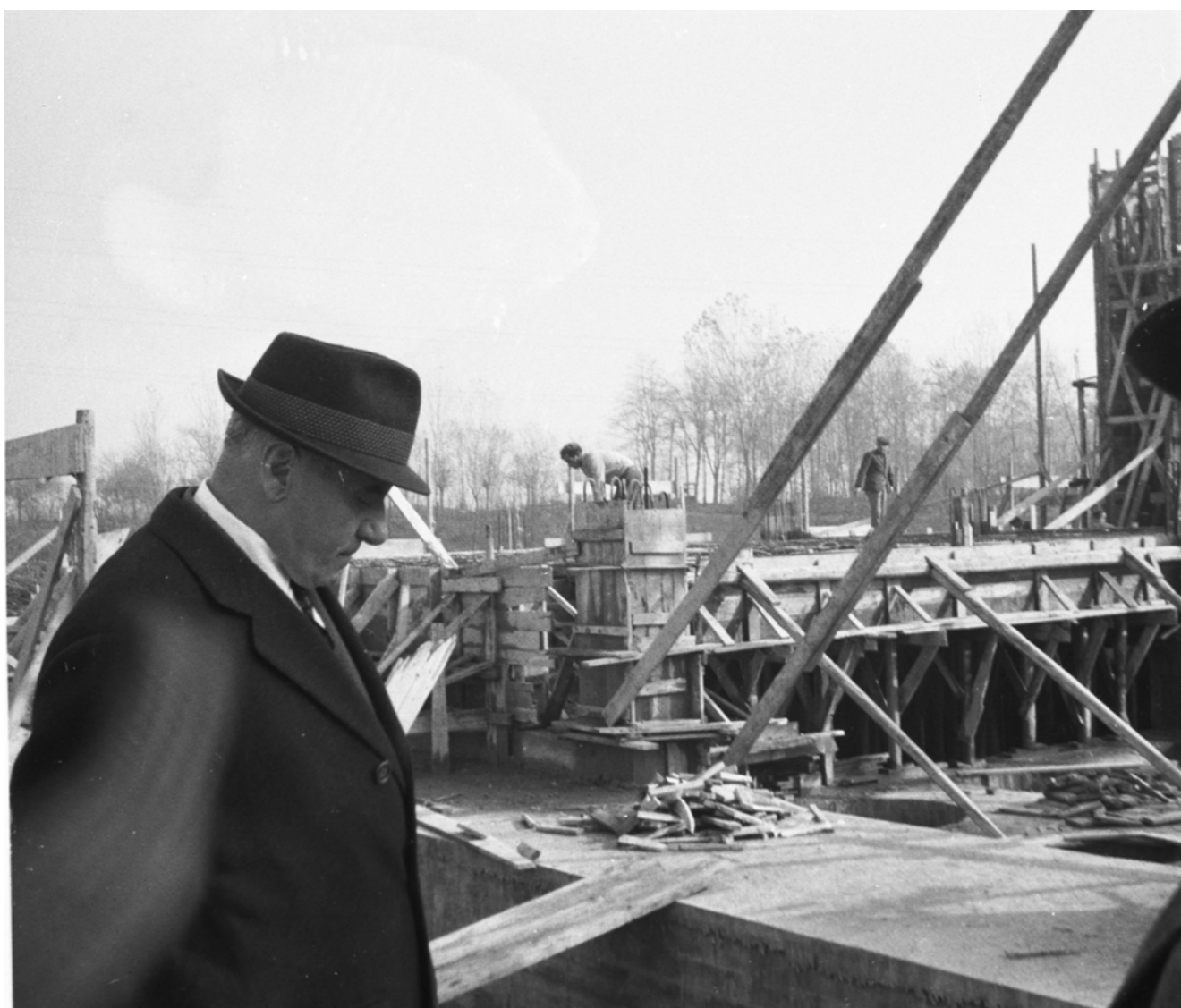
Beppe Lavazza at the construction site of the Strada Settimo factory, photograph, 1965
